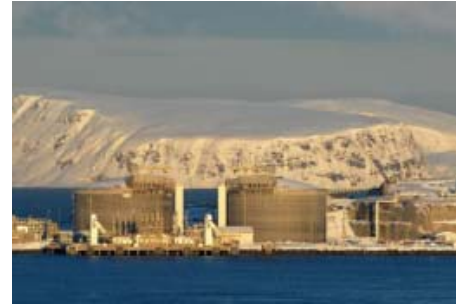
Snøhvit liquefaction plant, Norway
