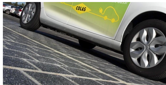
PV road (Colas) 13€/W
