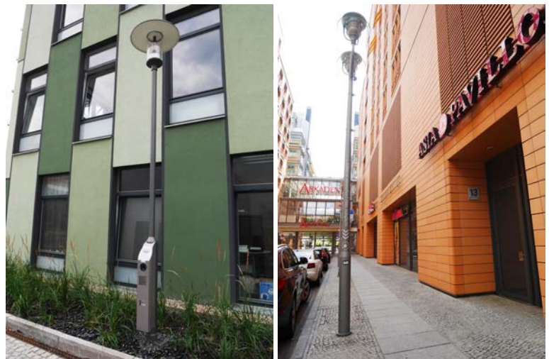
Combined street lighting and EV charging, experimented at INNOZ campus and Berlin City center © Photo LIAT
